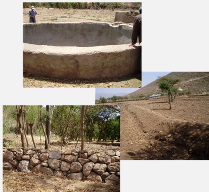
Figure 5. Types of soil and water conservation techniques applied in Boset Area (water ponds soil bunds, stone bunds, from up to down) (own source)
